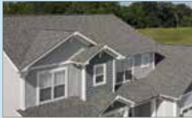
Roofing and Ventilation
